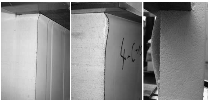
Figure 7: Failure modes at load application
