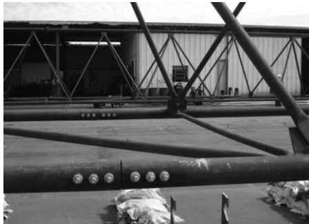
Figure 4: Tube sleeve connection.
