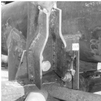
Figure 9: Diagonals reinforcements.
