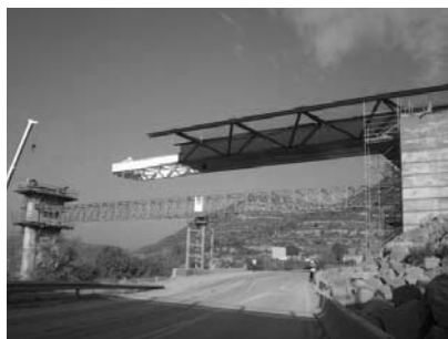
Figure 5: Launching the steel structure across the first two spans.
