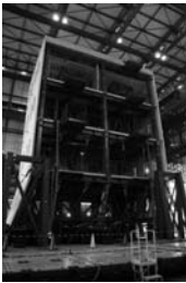
Figure 1: Collapse of the four-story steel building.
