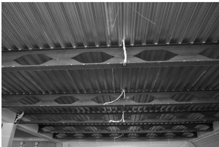
Figure 1: Thermocouples located at the midspan on the castellated beams and its connections
